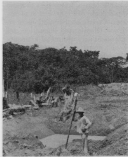
FIGURE 112.—In the Fundacion District of the Santa Marta Banana Region. Opening up a draining ditch for irrigation and drainage. Before the land is made ready for the ditch the heavy tropical hardwood forest must be cleared.
