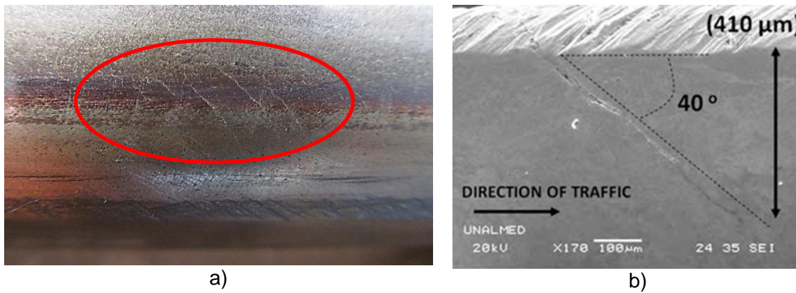
Figure 11. Rail fatigue damage: a) head checks, b) depth and crack angle with respect to the rail surface.
