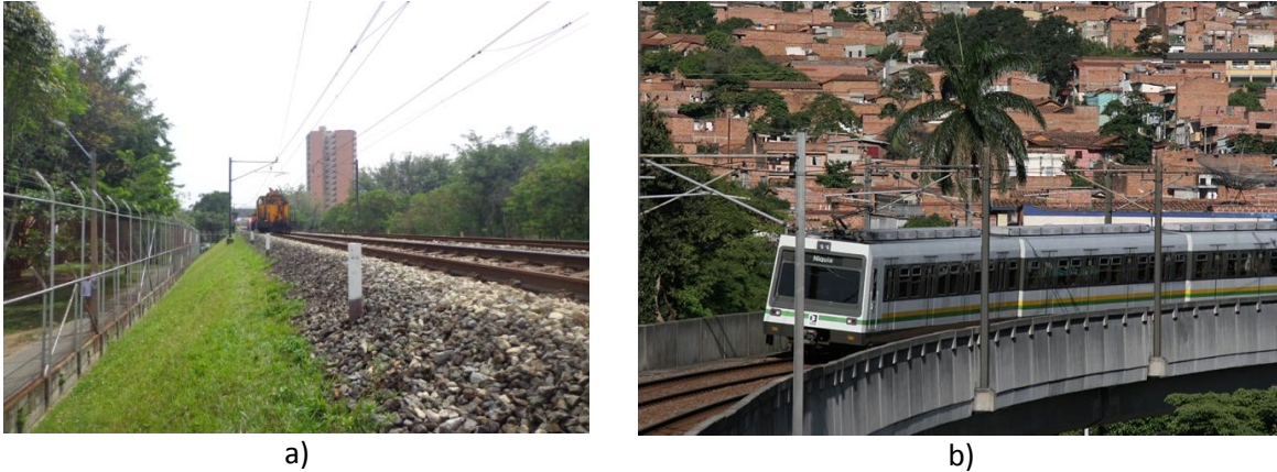
Figure 43. Metro of Medellin tracks. a) Not elevated track b) Elevated track.
