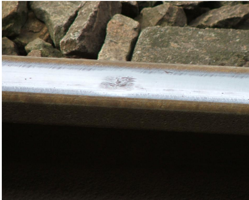
Figure 8. Burn mark on the top of the rail by adhesion loss.
