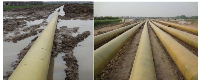
Figure 7. Photos of GFRER Protective Coating on Completion
