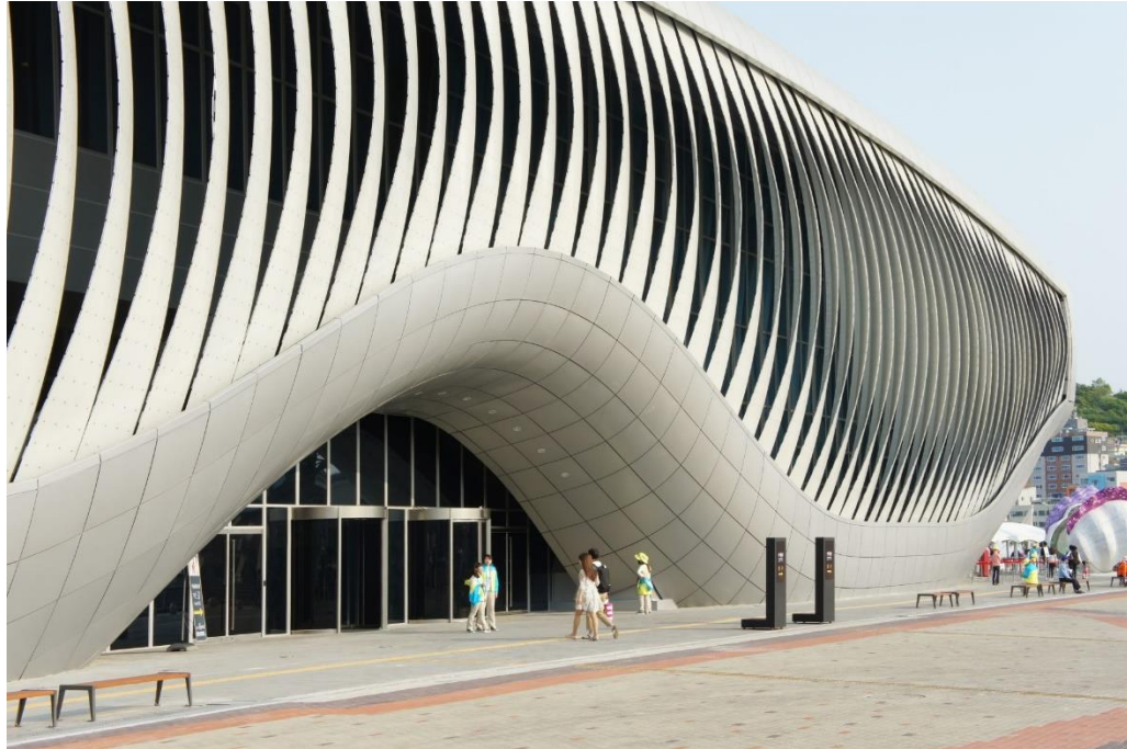
Fig. 12. One Ocean Theme Pavilion (Jeollanam-do) skin made of glass fiber reinforced polymer triggered by pneumatic actuators SOMA 2012
