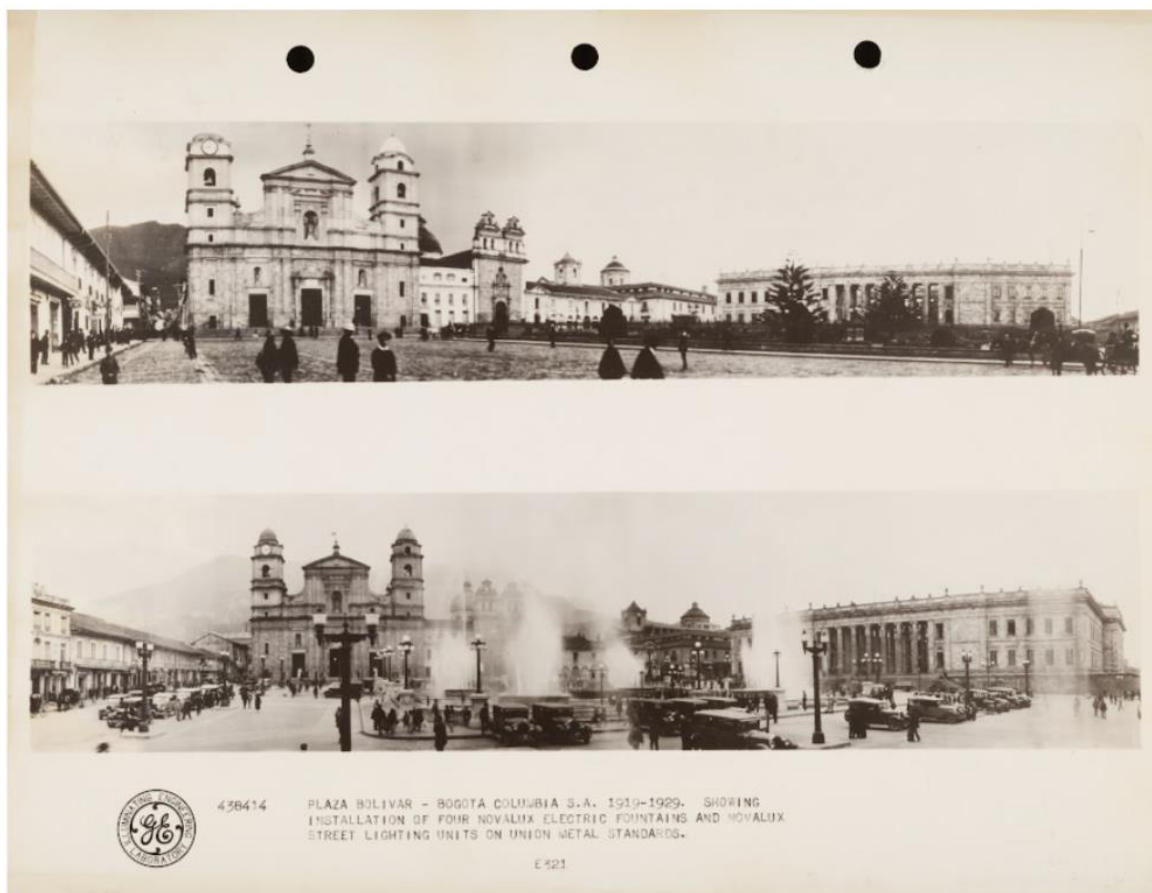
General Electric Company (1930). Plaza Bolívar - Bogotá Colombia S.A., 1919 - 1929. Showing installation of four Novalux electric fountains and Novalux street lighting units on Union Metal standards. Fotografía, 8 x 10 cm.
