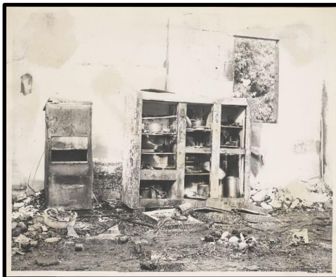
68 – UFC Ph. 30a, 1925-1955. Fire destroyed building 805-Sevilla Club and Mess on Feb. 25, 1955 midnight, March 10, 1955.
