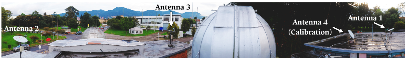
Figure 4-17.: Panoramic of the installed interferometer on the roof of Observatorio Astronómico Nacional - Campus building, Universidad Nacional de Colombia.
