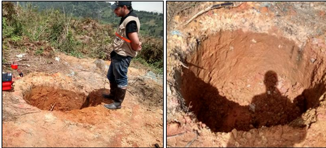
Figure 2-18: Test pit excavation. [From: Galeano (2020)].
