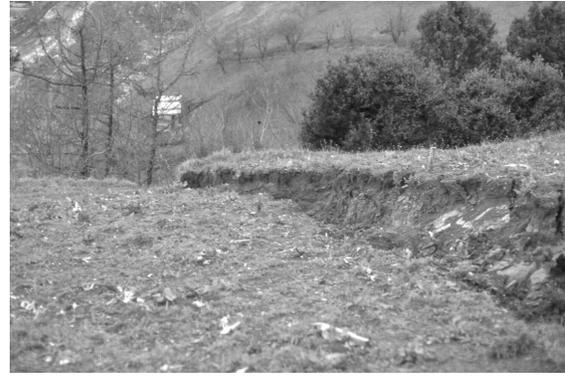
**Figure 9.** Picture of the tension crack in the upper part of the slope
