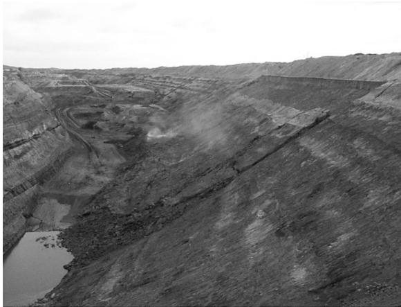
**Figure 11.** Picture of the footwall slope failure in Leigh Creek mine
